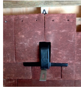
Step 3: Cut tiles around the hood of the SolarFlash as per page 12.
