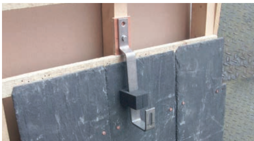
Step 1: Fix foam to bracket drop.
