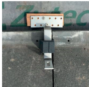
Step 2: Put SolarFlash (small) on the bracket.
