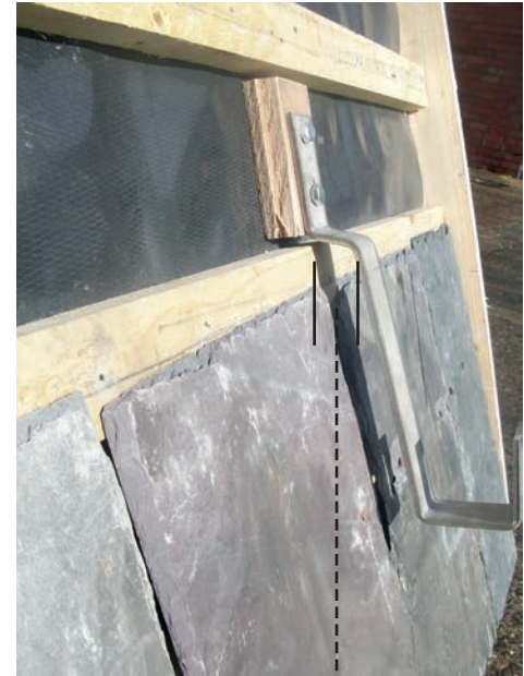
Slate roof showing 30mm clearance
