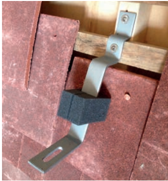
Step 1: Fix foam to the bracket drop.
